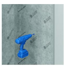
• Panels used to create walls for shower cabins and furnishing elements can be assembled using a hybrid sealant, such as Mapeflex MS45, and mechanical fasteners.
